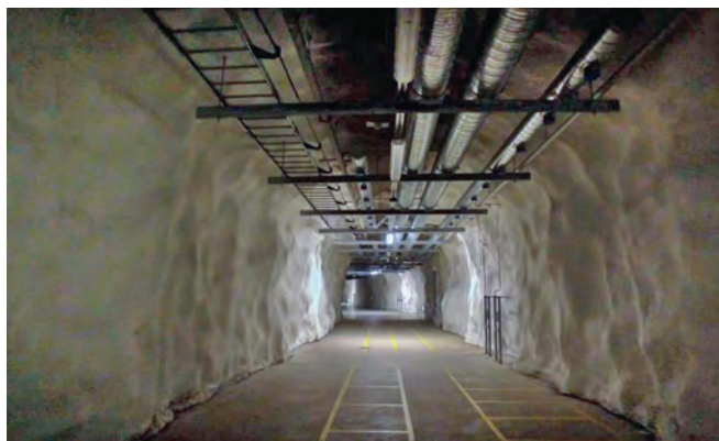
Part of the tunnel network under Helsinki
